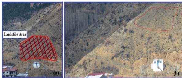
Figure 4.a) Close-up view and b) long-distance view of the main landslide mass.
