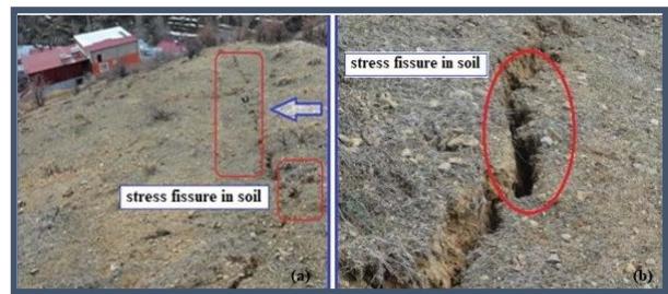
Figure 5.a) Distribution of stress cracks on the landslide mass. b) Wide-range stress cracks on the landslide mass
