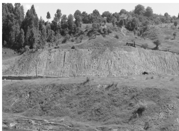
Figure 6. Sterile dump impacted by forms of erosion (Jieţ village)
