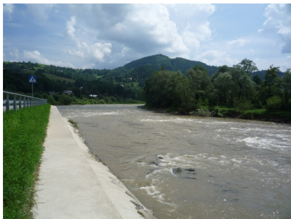
Figure 7. Cross section XI (km 19 + 870) with the strengthening of the right edge with a concrete wall (photo by M. Nawieśniak)
