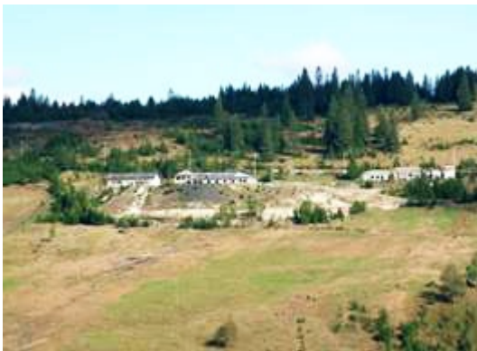
Figure 2. Mine in the Mestecaniș area ,6 th drift (General view)
