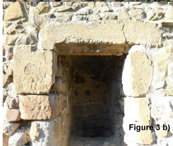
Figure 3. a. The sandstone lining of the Gothic window in wall of the chapel; b. the sandstone lining of the niche in the wall of the fortification
