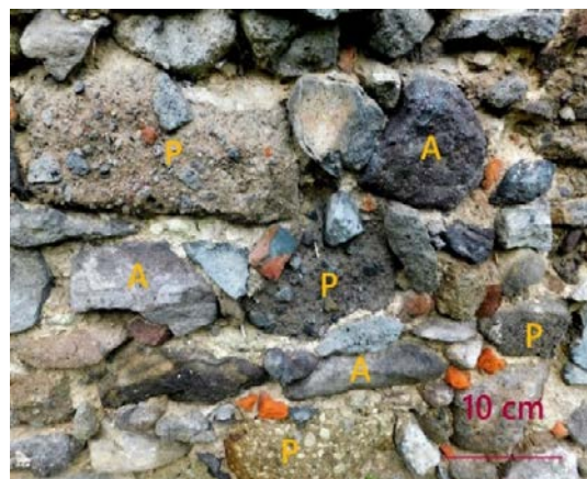
Figure 2. The wall of the cloister: andesites (A) and pyroclastic material (P)
