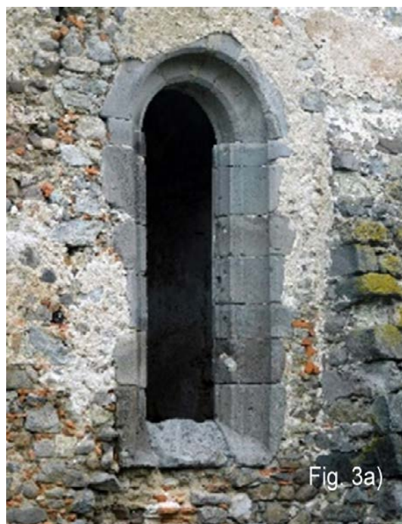
Figure 2. The wall of the cloister: andesites (A) and pyroclastic material (P)
