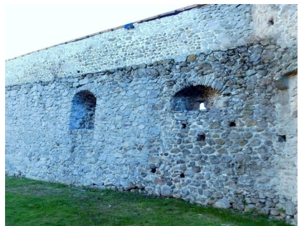
Figure 6. The fortification is built by andesitic rocks
