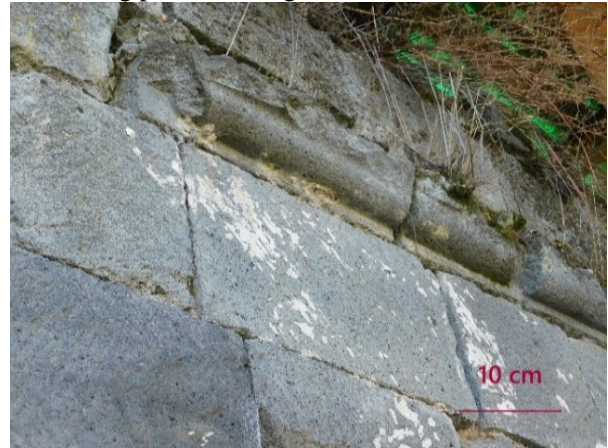
Figure 5. Details of the rest of a wall of the Cistercian Abbey built from carved pyroclastic rocks
