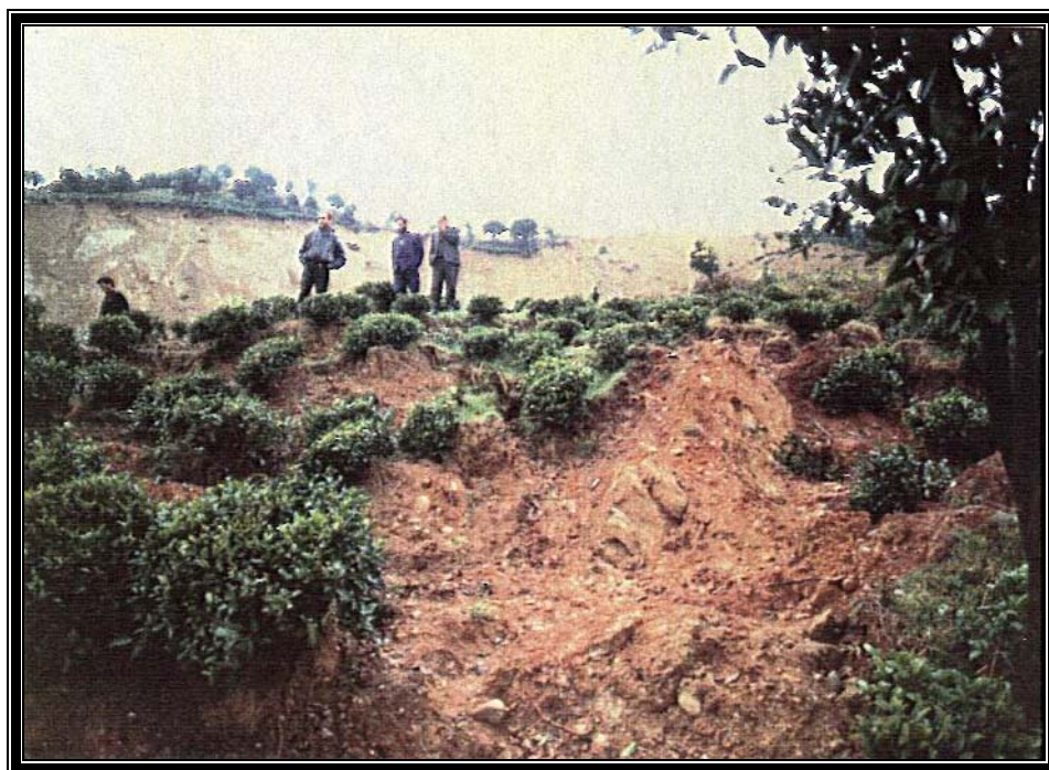
Figure 9. Destruction due to landslide in a tea garden.
