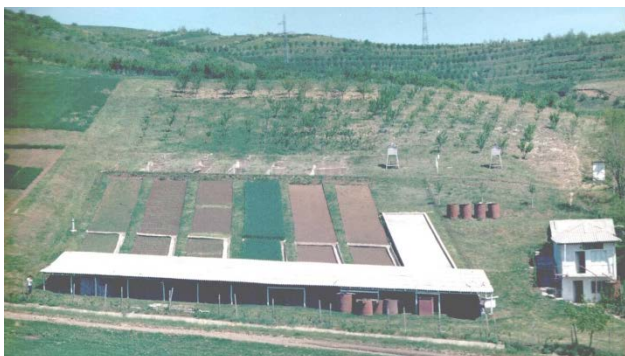
Figure 3. General view of the Research Station for Soil Erosion - Aldeni, Slănic-Buzău River Basin
